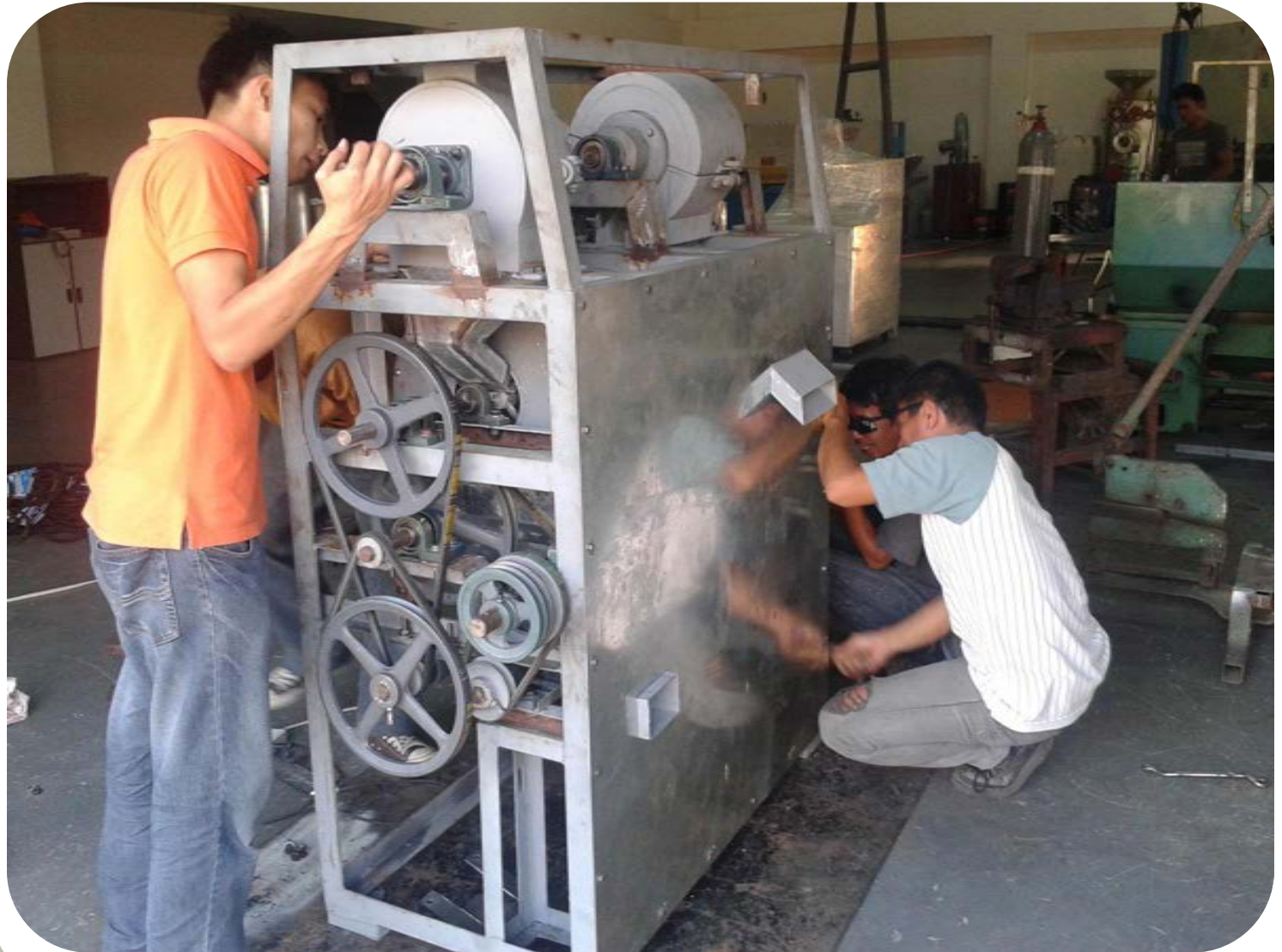
Fabrication of the cornmill machine incorporating the different design of each cornmill component
