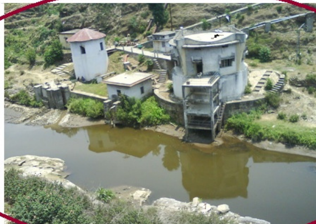
Kosi Pump House
